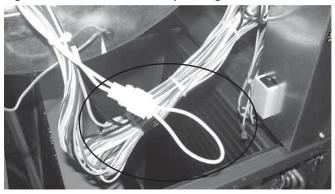
Note: For 115v power only. Damage will occur to motor with 230v power supply if 115v jumper is used.
