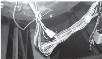
Figure 10: Install Two Pin Jumper Plug
